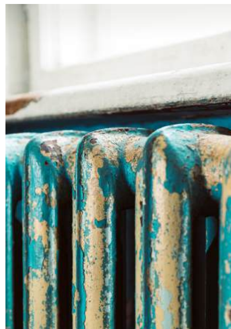
Peeling lead paint in older buildings, as shown on the radiator above, is among the health hazards Women for a Healthy Environment has been targeting since its inception. Its work has included advocating for legislative remedies such as the Pittsburgh Lead Safety Law, which calls for addressing the ways people, especially children, are exposed to lead hazards.
